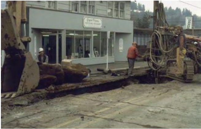
Image of 17-foot-deep trench line for sewer separation on High Street in Oregon City, Oregon. Picture windows of business are less than 10 feet away.
