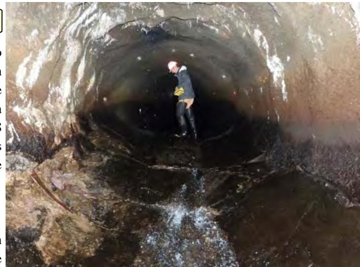
Photo: Spirit Lake Tunnel April 2014. Invert of the tunnel has heaved up 2.4 feet decreasing the hydraulic capacity of the outlet tunnel.
