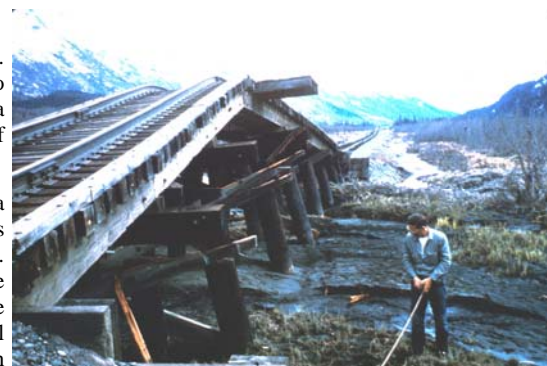
A graphic example of how the 1964 Alaska earthquake caused damage by means of lateral spreading toward channels
