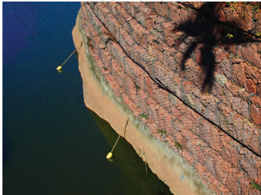
Gabion Basket Wall used for Mexican Iguana Habitat Restoration
