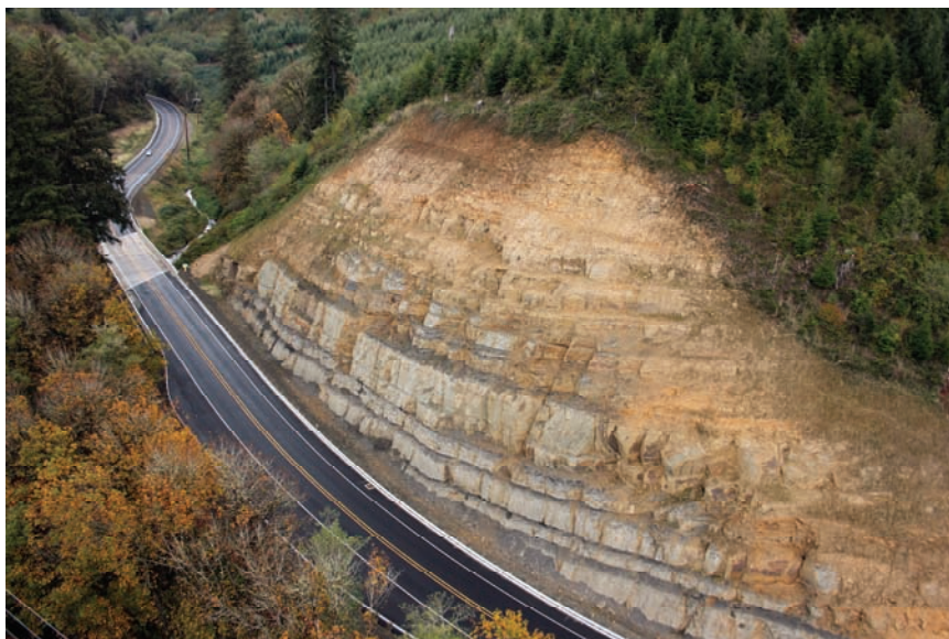
View north along US 20 showing Tyee Formation sandstone and siltstone exposed in new cutslope adjacent Simpson Creek Bridge.
