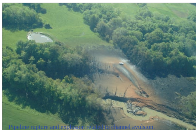
Pipeline rupture and explosion related to channel avulsion.
