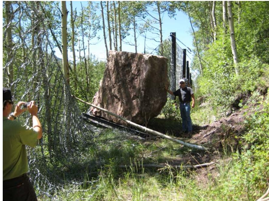
The October photo is from Steve Mumma from the Geobrugg. This photo is of an August 2007 impact on a 12' high, 180 ft-ton design energy rockfall barrier installed at a residential development in Telluride, CO. The boulder shown is approximately 40 tons and originated from a cliff up-slope of the barrier. The boulder rolled down the slope, leaving a trough in the ground and a path of flattened trees before being stopped by the rockfall barrier.
