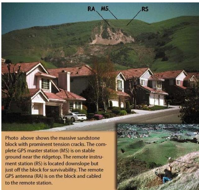
Photo above shows the massive sandstone block with prominent tension cracks. The complete GPS master station (MS) is on stable ground near the ridgetop. The remote instrument station (RS) is located downslope but just off the block for survivability. The remote GPS antenna (RA) is on the block and cabled to the remote station.
