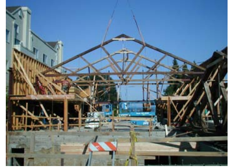
Installation of reused roof trusses during construction
